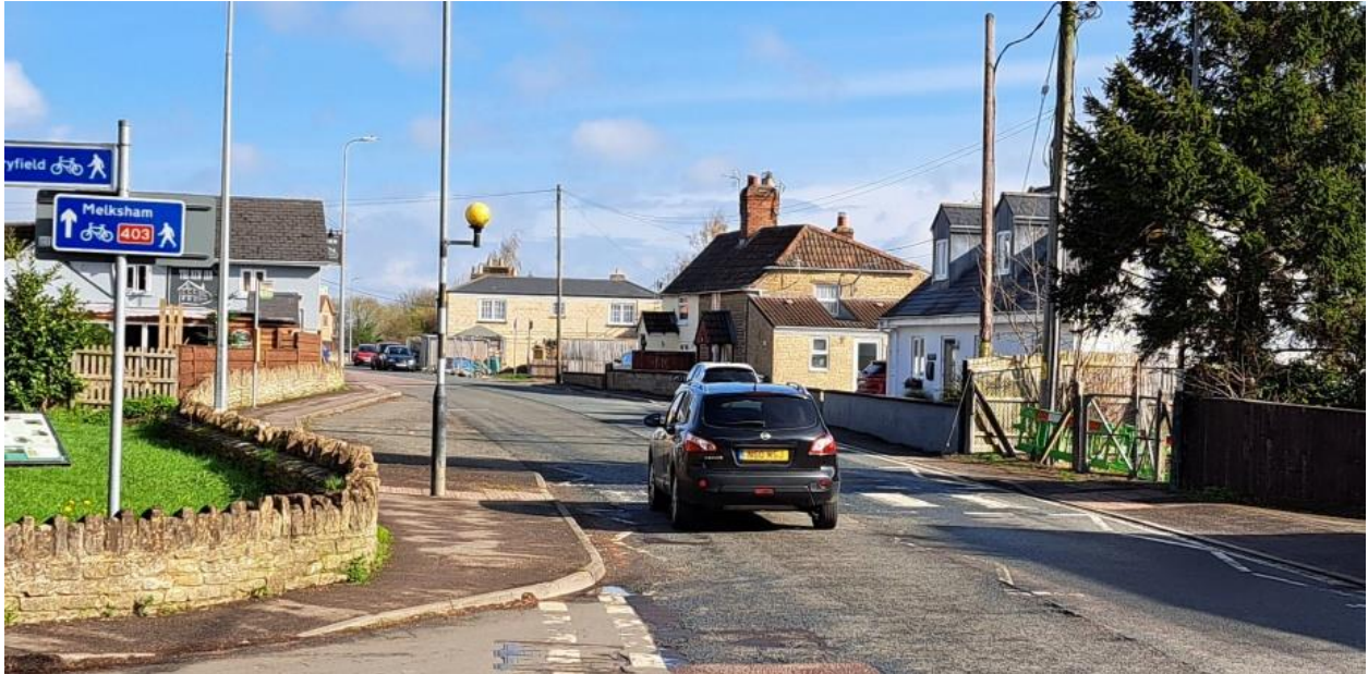
Semington Road – north of access - location of proposed new cantilever bus stop (left) and new zebra crossing road marking.
